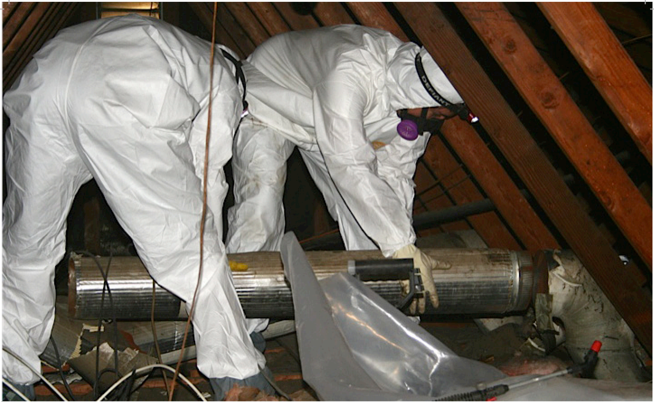
DUCTS ARE DISCONNECTED AND LIFTED OUT OF THE TOP OF THE FURNACE AND REGISTER BOOTS
